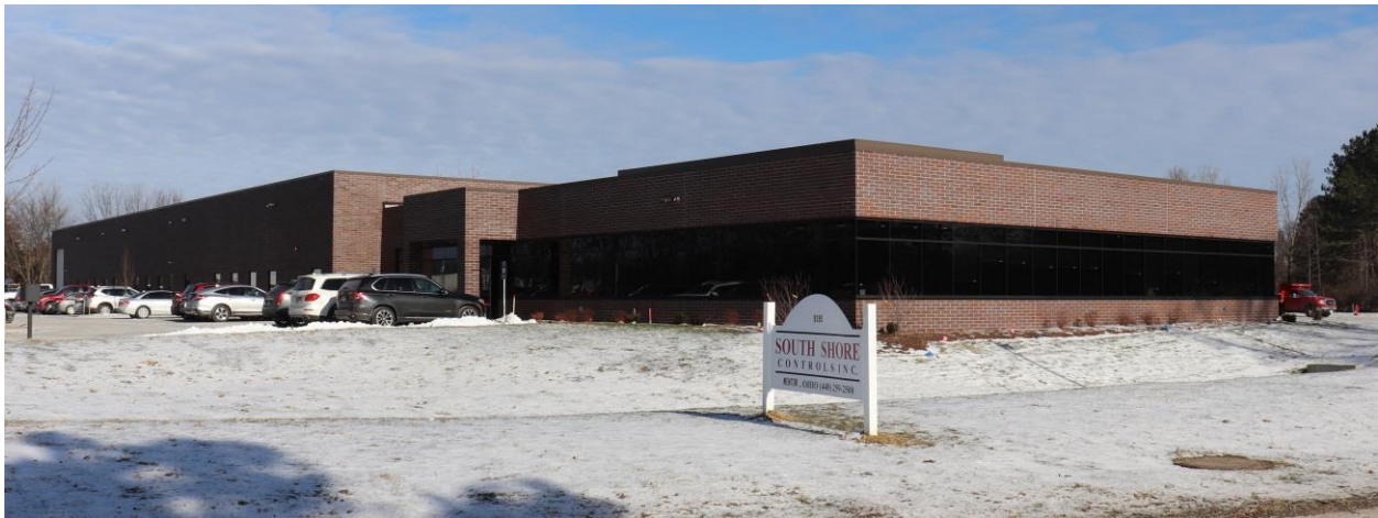
South Shore Controls and Niagara Systems - New Headquarters - Mentor, OH
